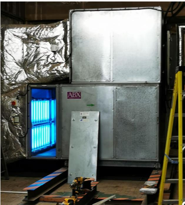
This provided a cost-effective solution to the air quality in the area, the arrays were wired back to the air system's control panel, so they only came on when the air was recycled.
